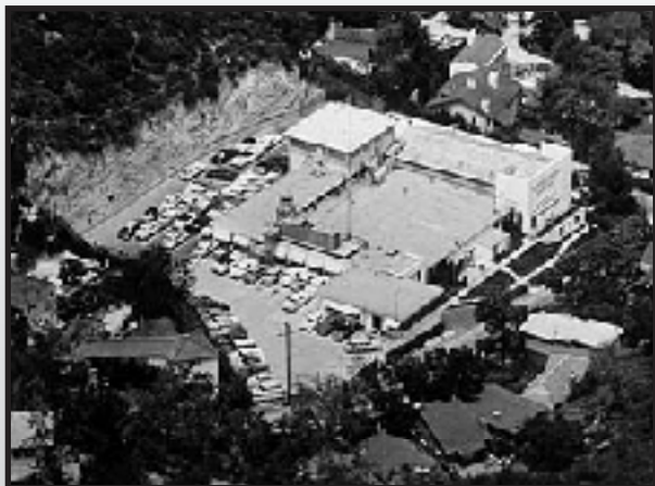
The Lookout Mountain facility was a fully self-contained 100,000-square-foot studio overlooking the famous Sunset Strip.
