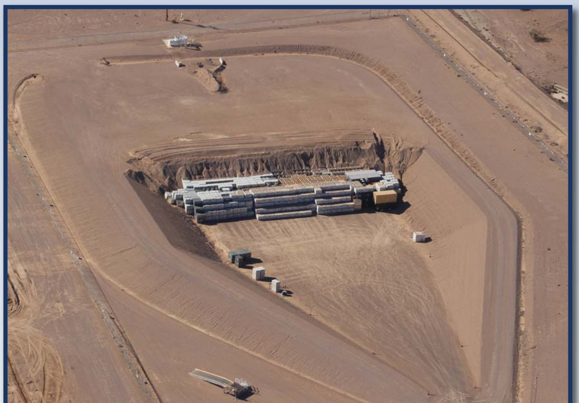
MLLW Disposal Cell at the NNSS Area 5 Radioactive Waste Management Complex (partially filled in October 2015)
