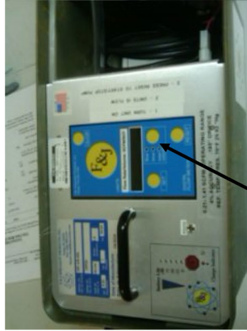
Flow/time/total volume indication button Make sure Flow is showing.
