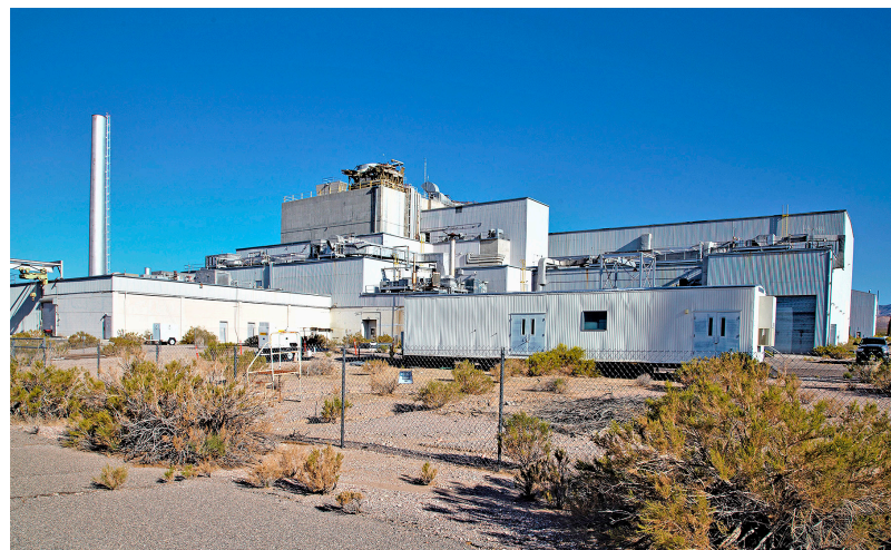
Characterization is underway in preparation for demolition and closure of the EMAD facility.
