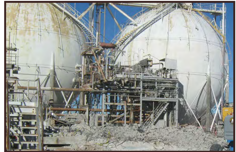
Ancillary structures at Test Cell C
