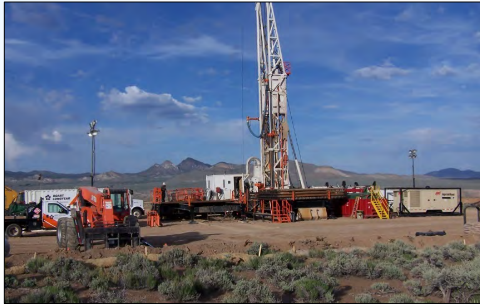
Installing new monitoring well at CNTA
