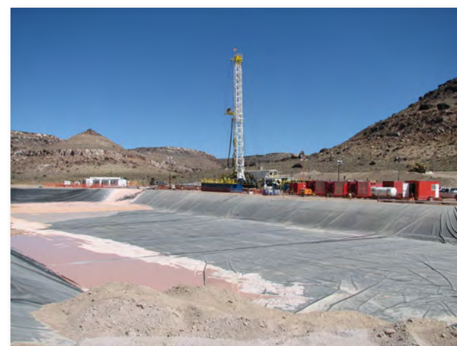
Lined Sump at ER-EC-11 to Hold Up to Four Million Gallons of Water During Well Drilling & Pumping Activities
