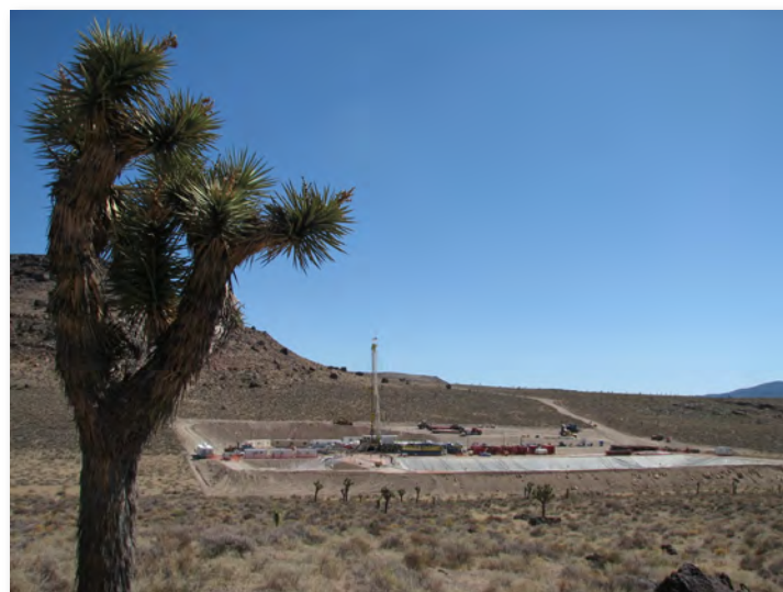
Well ER-EC-11 During Drilling
