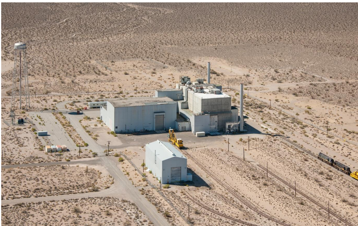
Figure A-28. The NRDS Engine Maintenance and Disassembly Building (photo taken by Remote Sensing Laboratory 2013)
