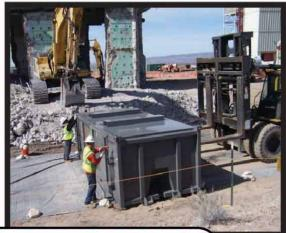
Workers use specialized equipment and methods to demolish large buildings so that radioactively contaminated debris can be packaged for disposal.
