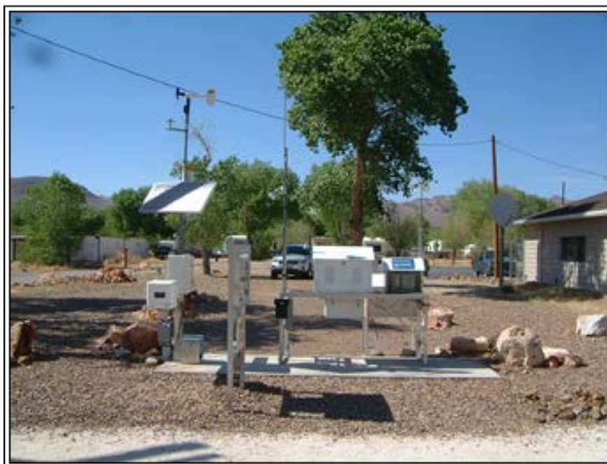
Figure 7-2. CEMP Station in Betty, Nevada
