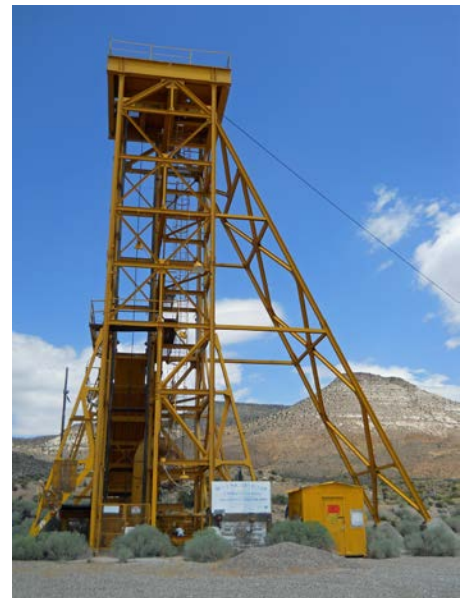
Figure 14-1. Structural frame above the main shaft to the underground U15 Complex.
