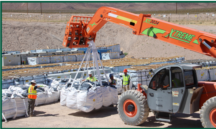
Waste cells are put in a 20' x 20' grid system, using letters and numbers to mark the location of waste packages.
