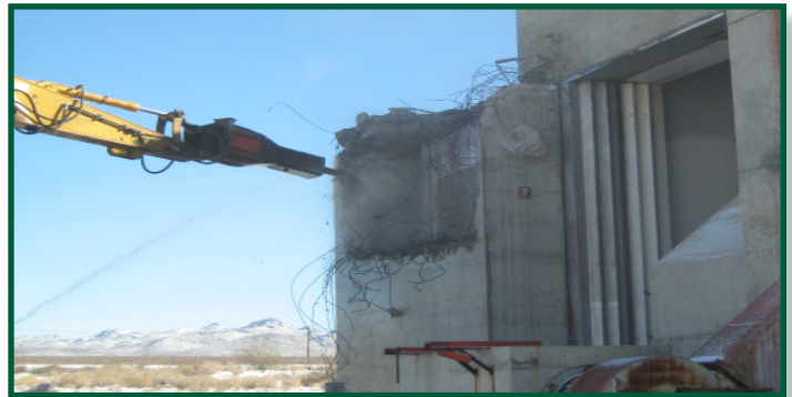
Demolition work at R-MAD using a hydraulic hammer
