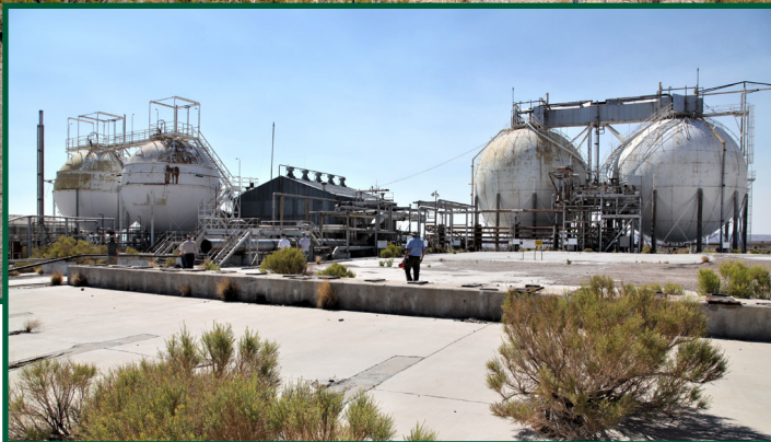
Test Cell C
