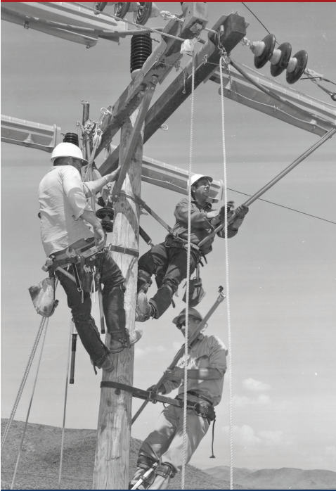
Crew working on one of the lower-energy distribution lines in Frenchman Flat. Most of the distribution lines used single pole structures while the 138 kV line was supported by wooden H-frame structures with cross bracing. (REECO neg. 3217-9 August 1970).
