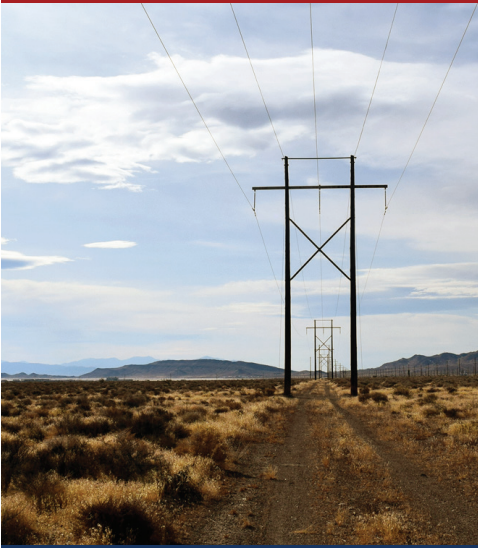
The original wooden towers of the 138-kV transmission line stand as silent sentinels across the Cold War landscape that once was the site of atmospheric and underground nuclear tests (Photo: DSC_0026, DRI November 2020).
