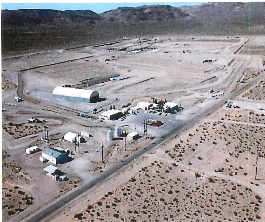
Figure 5 – Area 5 Radioactive Waste Management Site
