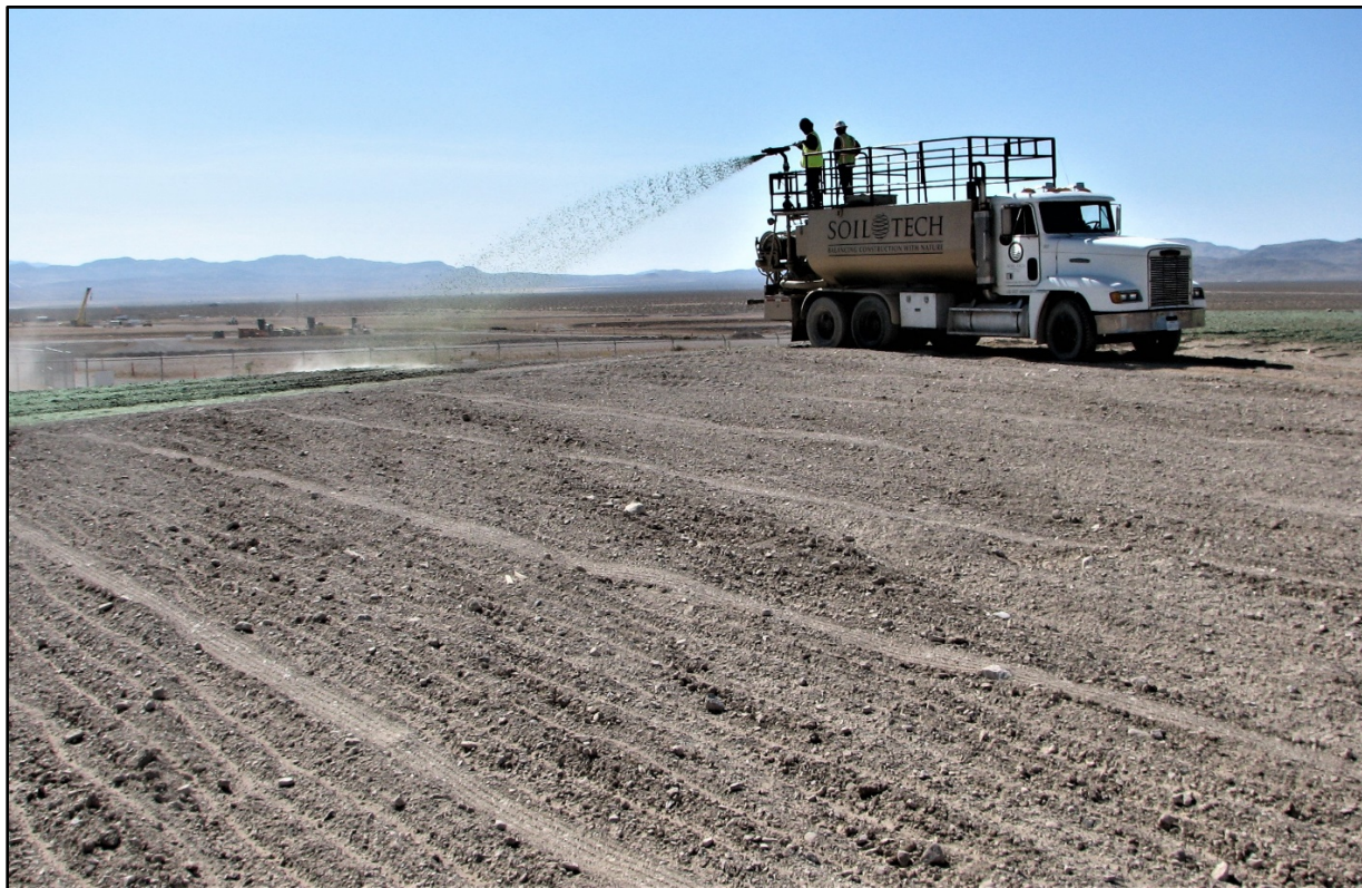
Figure 7-4. Applying hydromulch at the Cell 18 Cover Cap.
