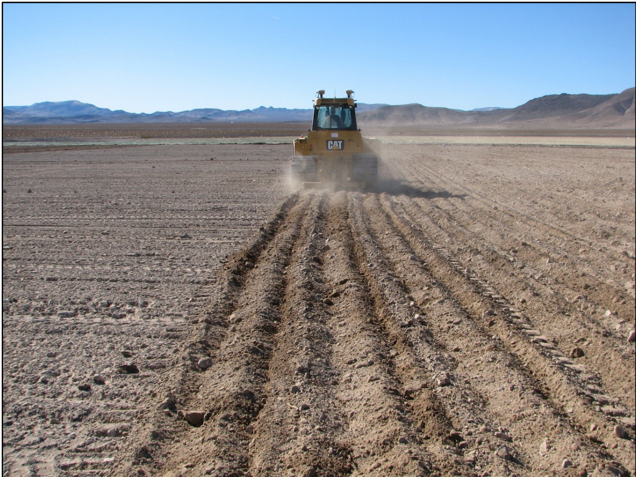
Figure 7-3. Ripping CAU 577 East Cover Cap with bulldozer to alleviate soil compaction.
