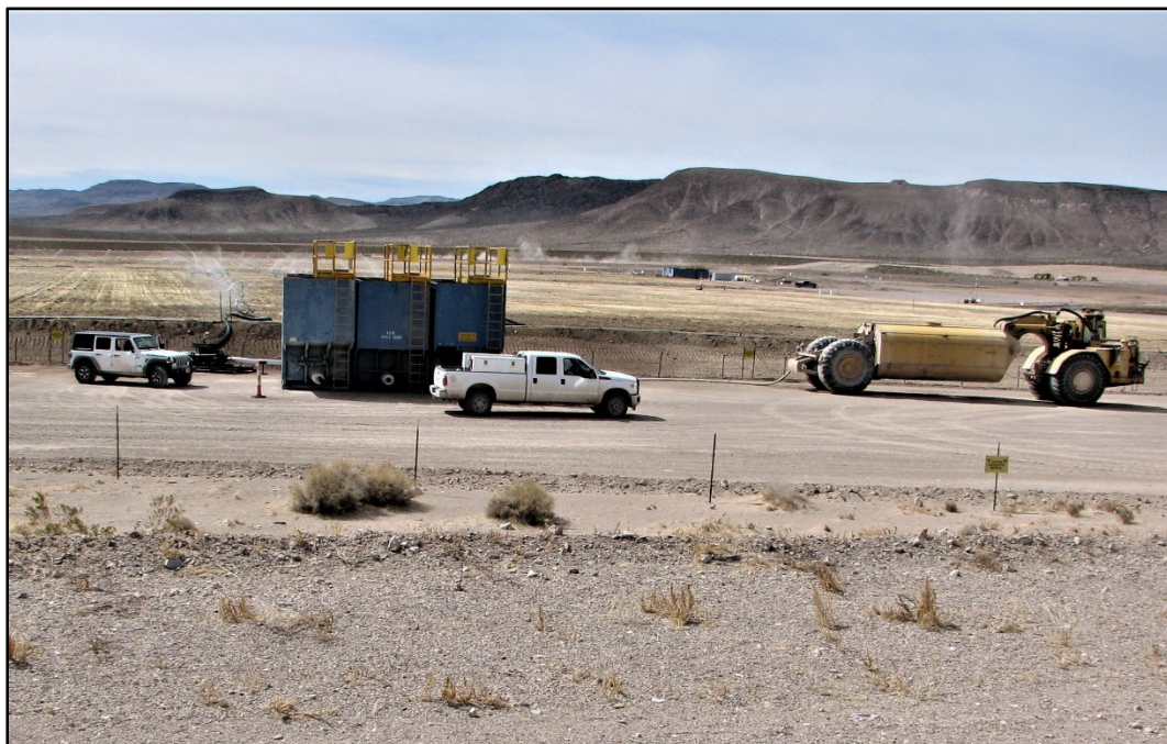
Figure 7-7. Watermaster filling water tanks at CAU 577 East Cover Cap.
