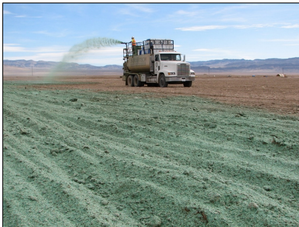
Figure 7-5. Applying hydromulch on CAU 577 West Cover Cap.
