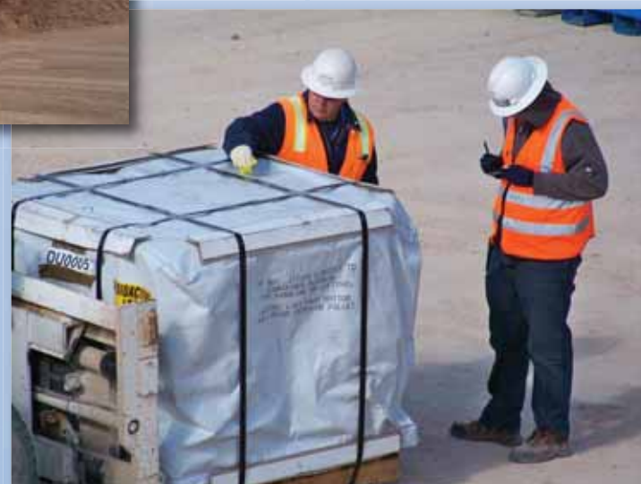
Workers conduct a radiological survey of a waste package prior to disposal in an excavated disposal cell at the NNSS Area 5 Radioactive Waste Management Site
