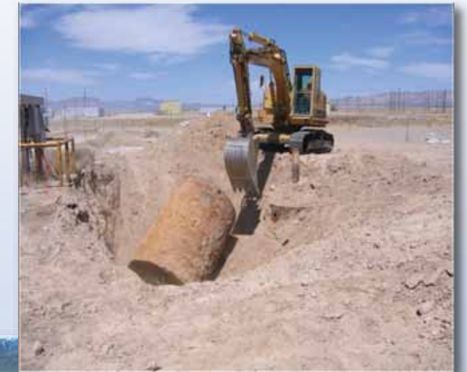
Tank excavation at the Nevada National Security Site
