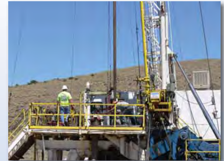
Crews drill a groundwater characterization well at the NNSS
