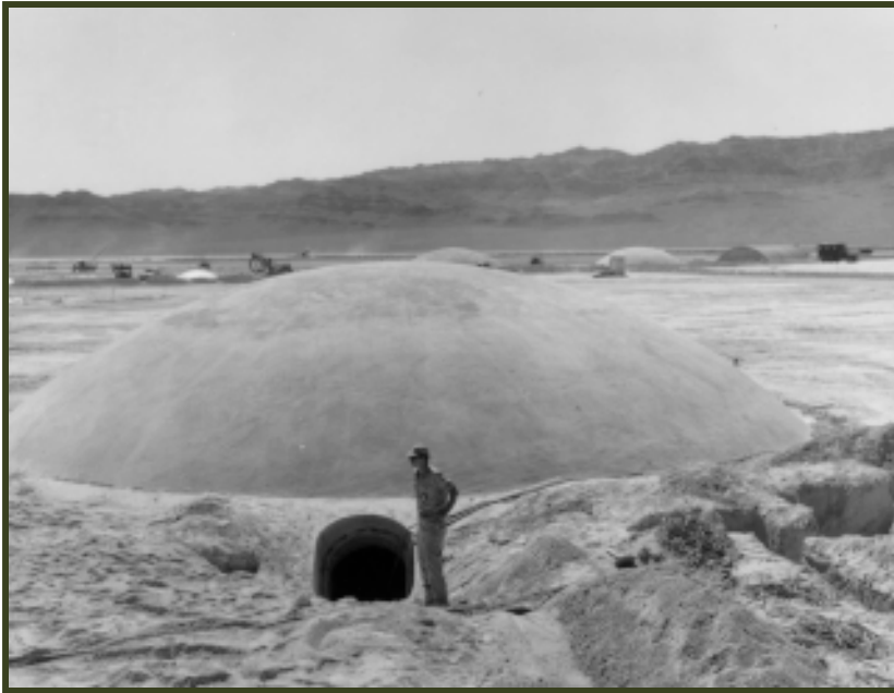
Concrete shelter domes prior to the 1957 Priscilla test
