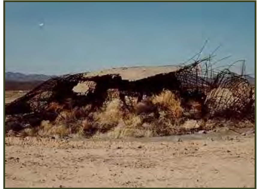
Effect of the test on the concrete shelter dome
