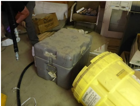
Second floor mezzanine, Density Gauge
