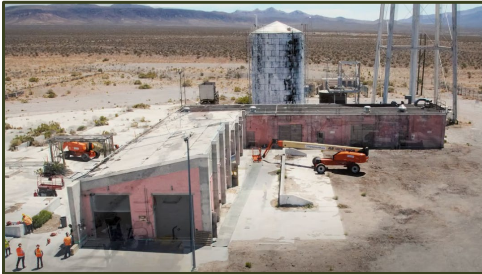
TCC Demolition Update - Before
