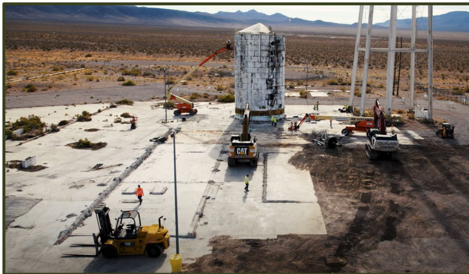
TCC Demolition Update – After
