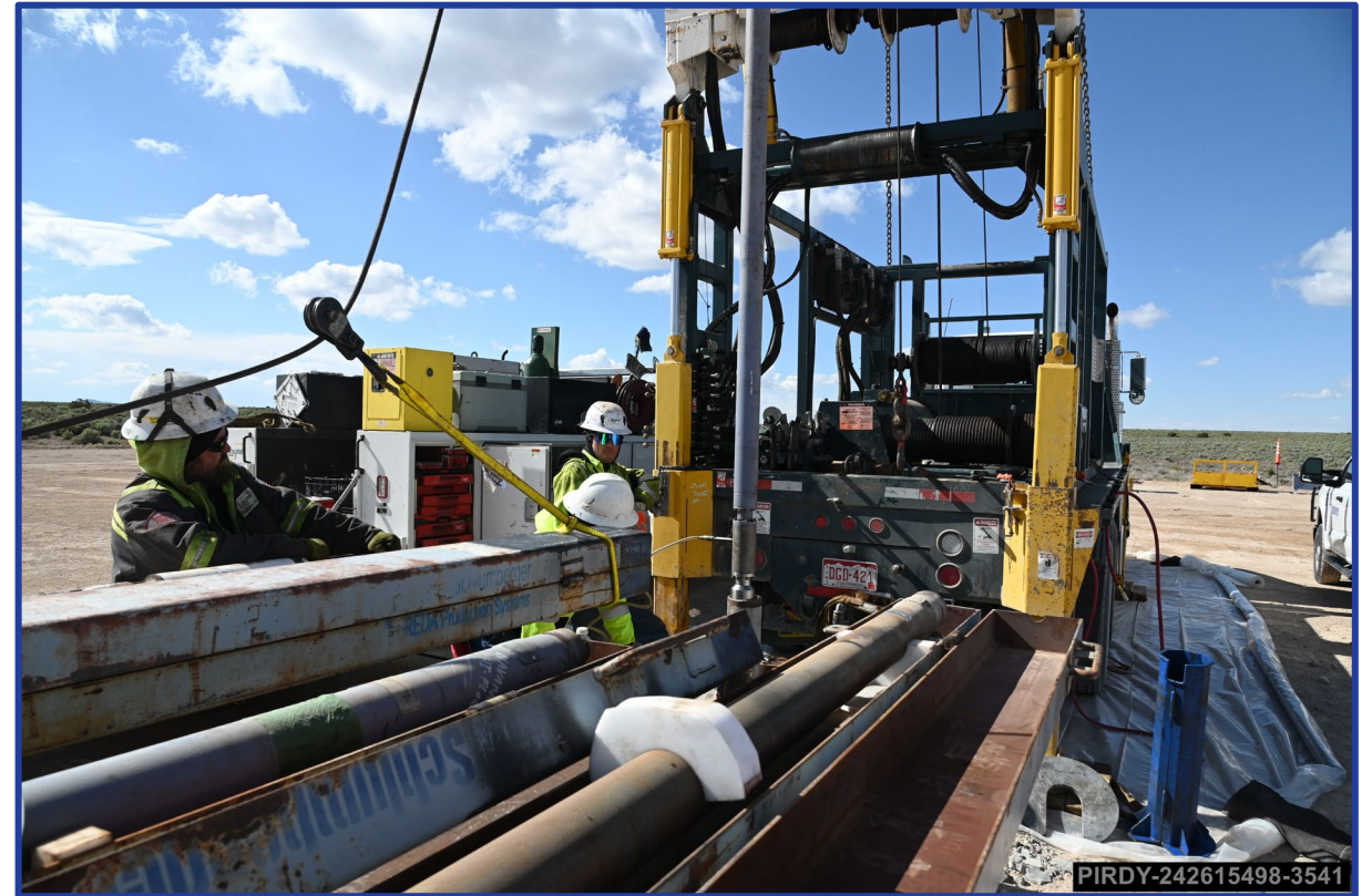
Pump Being Installed at ER-20-1 (May 4-8)
