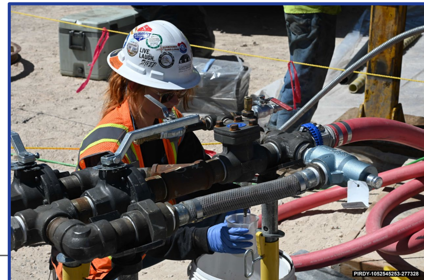
Obtaining Water Quality Sample at ER-20-1 (May 4-8)
