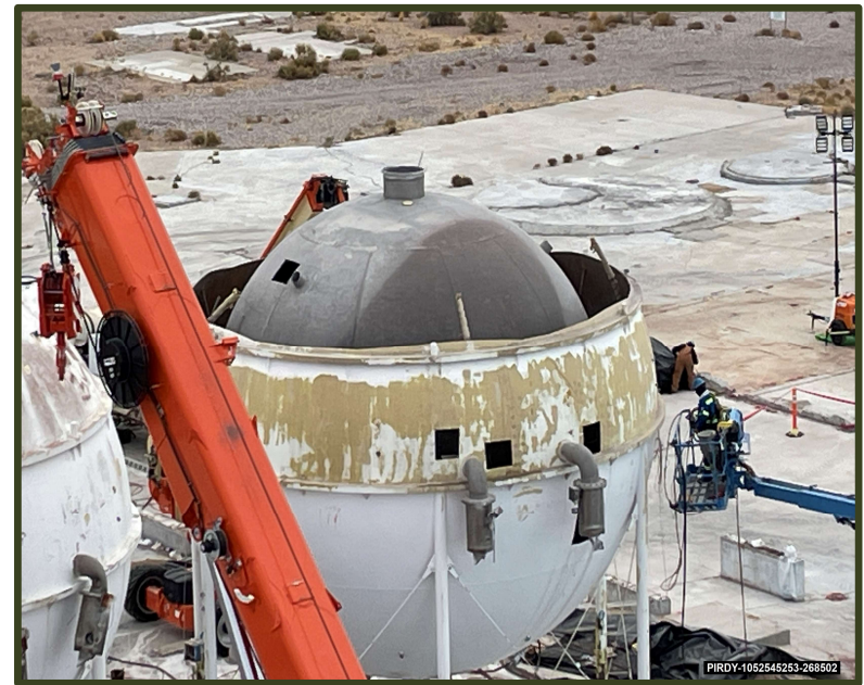
Dismantling of Dewar at Test Cell C
