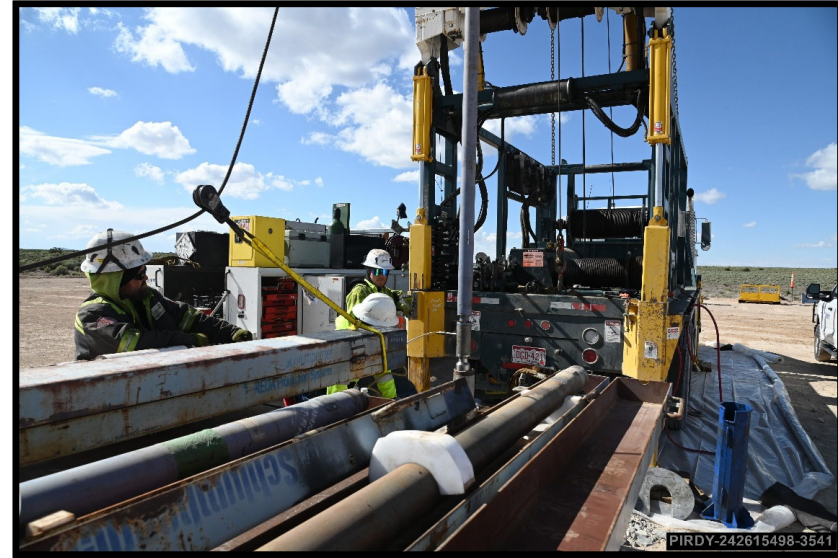
Pump being installed at ER-20-1 – May 2026
