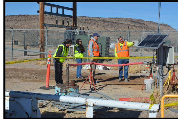
NSSAB observed groundwater monitoring at Well WW-C1 – March 2025
