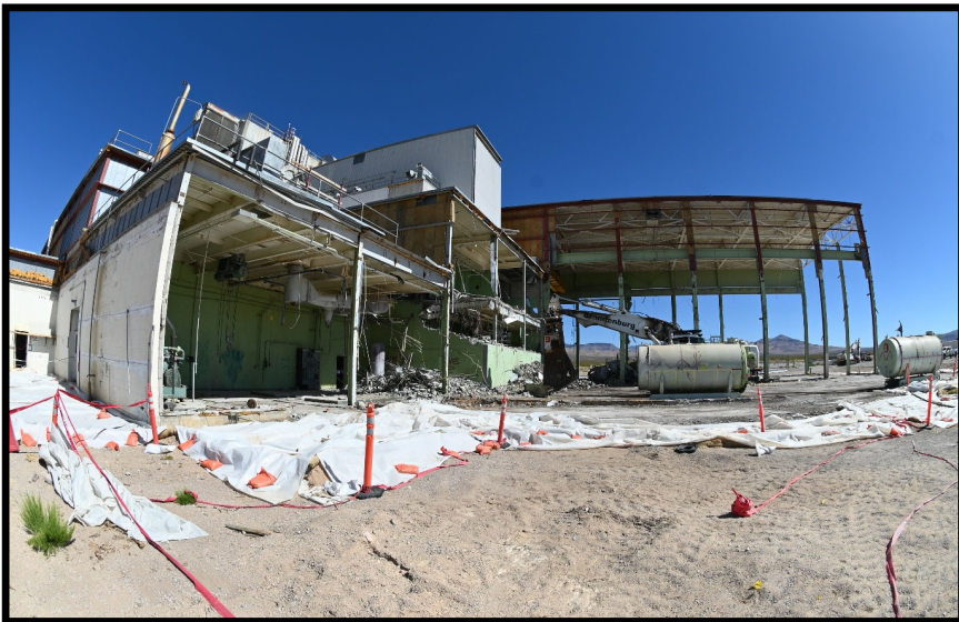
EMAD demolition progress on EMAD APFA – June 2026
