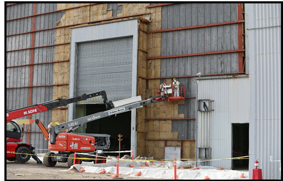
Galbestos removal at EMAD APFA – March 2026
