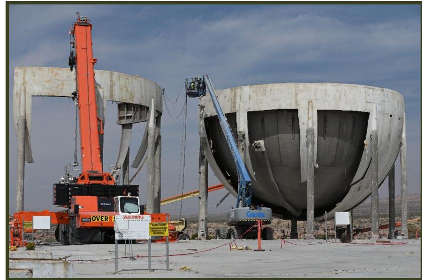
Hydrojet activities on the lower shells of Dewars 1 and 2 at Test Cell C
