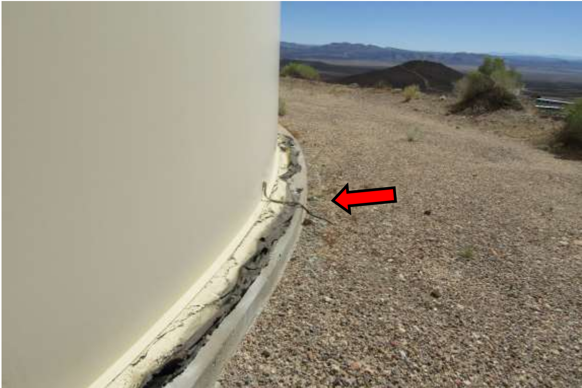
Photo shows the tank is electrically grounded for lightning protection as required by OSH Act of 1970 Section 5 and appears to be in good condition.
