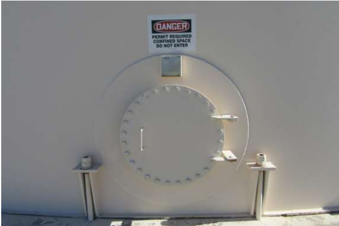
Photo shows the condition of the 24" primary shell manway, which is in compliance with AWWA D100-11; 7.4.4 Shell manholes, 14.7.2.1.1, NFPA 22-2018; 14.7.2.1.1 and OSHA 1910.146(c)(2) Confined spaces .
