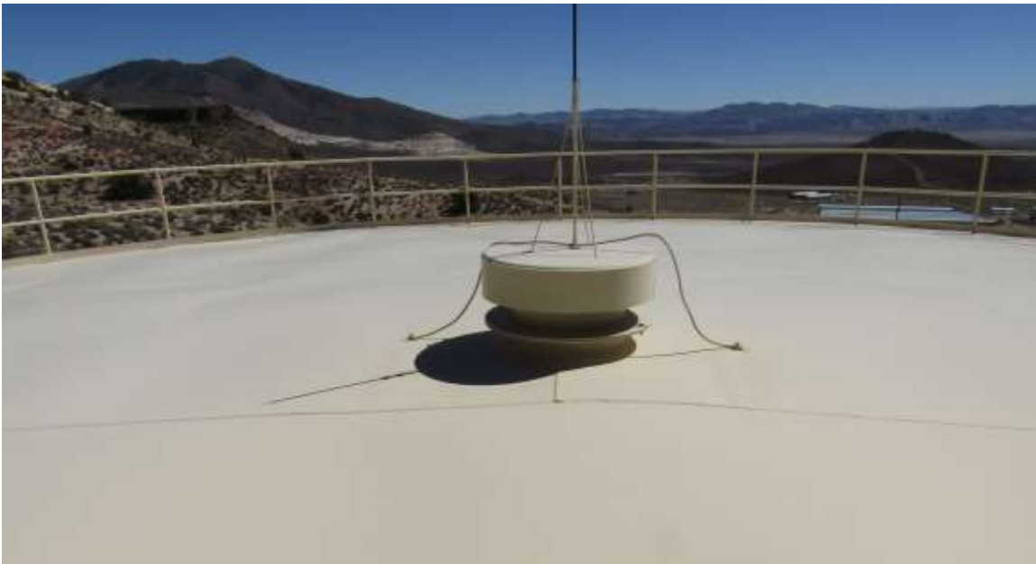
Photos show the existing roof vent, which appears to be in good condition.
