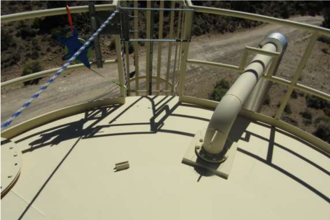
Photo shows the tank roof edge is equipped with a 43" high compliant handrail system for fall protection as required by OSHA 1910.28(b)(1) . The handrail system is equipped with an intermediate rail and toeboard.
