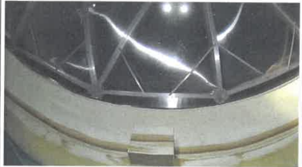
00:54 - Sediment staining on shell in fluctuation zone
