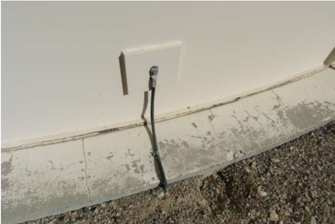
Photo shows the tank is electrically grounded for lightning protection as required by OSH Act of 1970 Section 5 and NFPA 780-2017; 5.4 Metal Towers and Tanks and appears to be in good condition.
