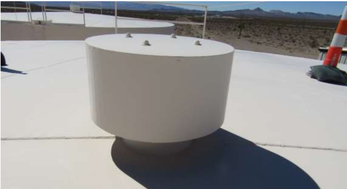
Photos show the existing 8" roof vent, which appears to be in good condition.
