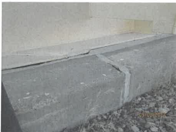
16 - Foundation grouting separating
