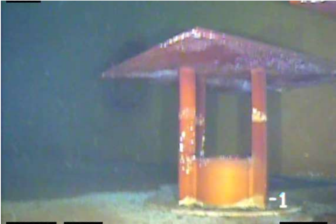
Photo shows a suction pipe on the interior of the tank, which is equipped with a properly sized anti-vortex plate to prevent formation of a vortex.
