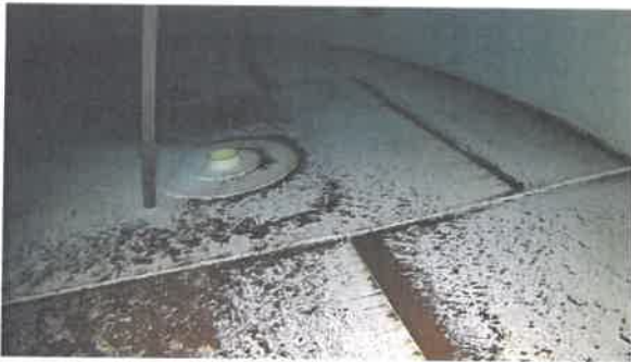
6:56 - Floor inlet pipe with sediment ring
