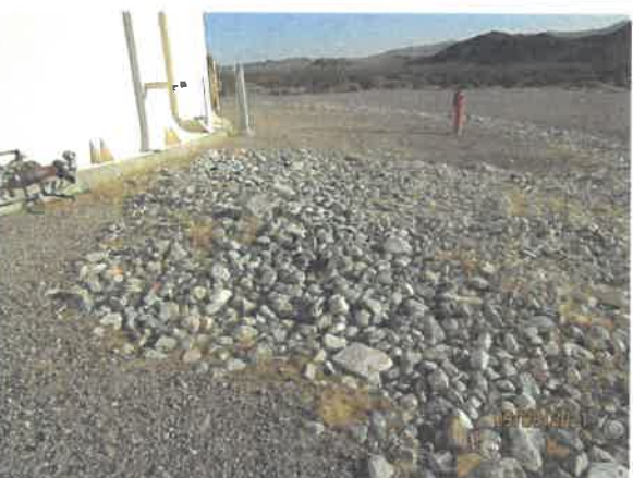
3 - Overflow discharge onto rocks
