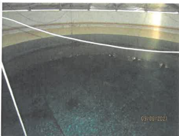
38 - Hanging cathodic protection system
