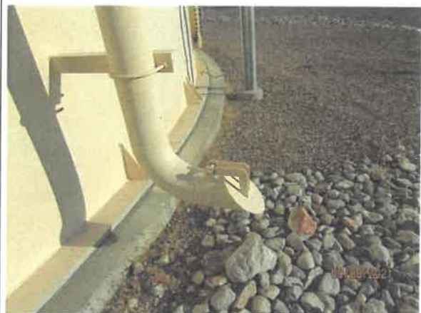
4 - Overflow with flapper valve
