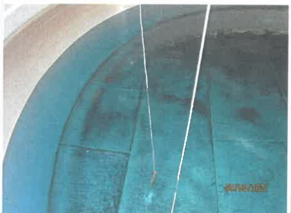
37 - Tank walls and floor, with hanging cathodic protection system
