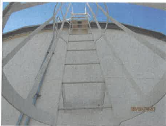
14 - Upper tank ladder with safety cage
