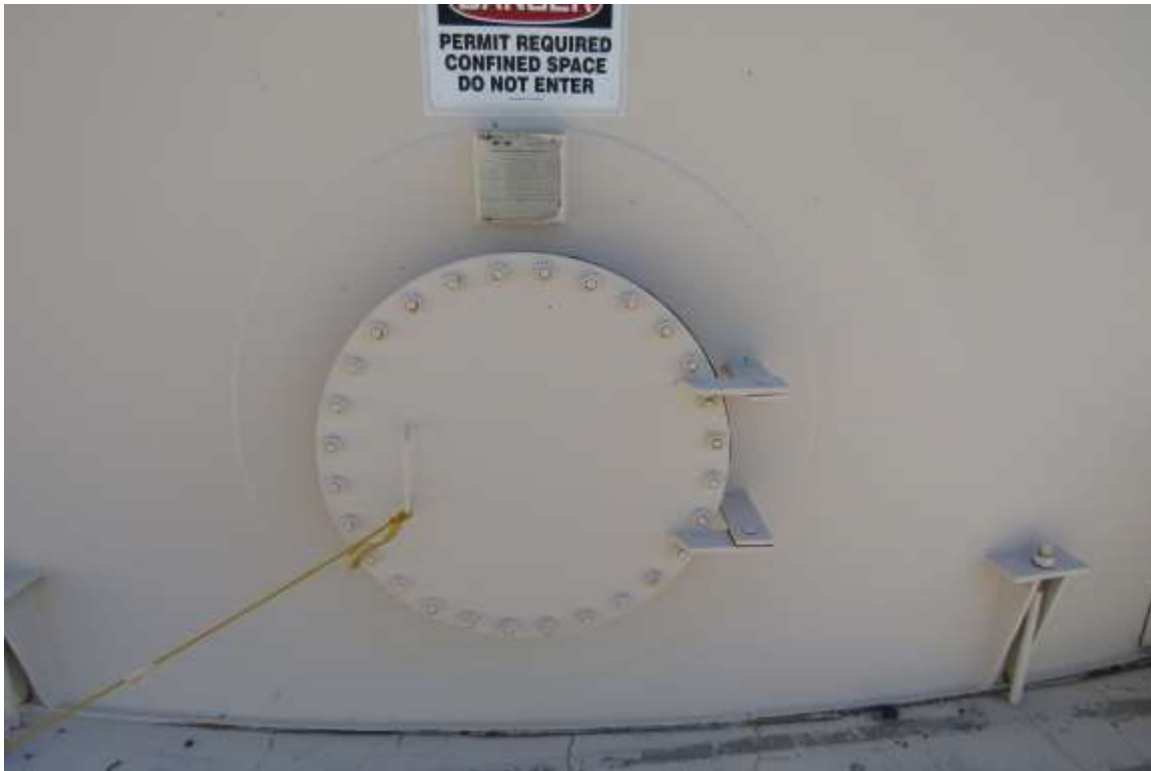
Photo shows the condition of the 24" primary shell manway, which is in compliance with AWWA D100-11; 7.4.4 Shell manholes , NFPA 22-2018; 14.7.2.1.1 and OSHA 1910.146(c)(2) Confined spaces .
