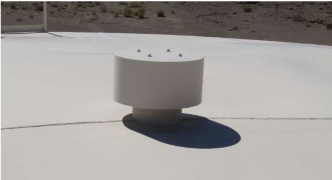
Photos show the existing 12" roof vent, which appears to be in good condition.
