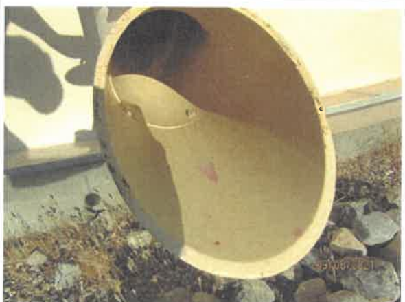
5 - Interior overflow pipe with no screen
