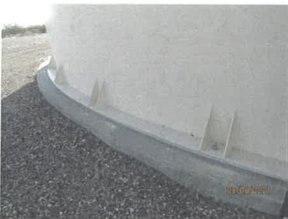
15 - Tank foundation typical condition
