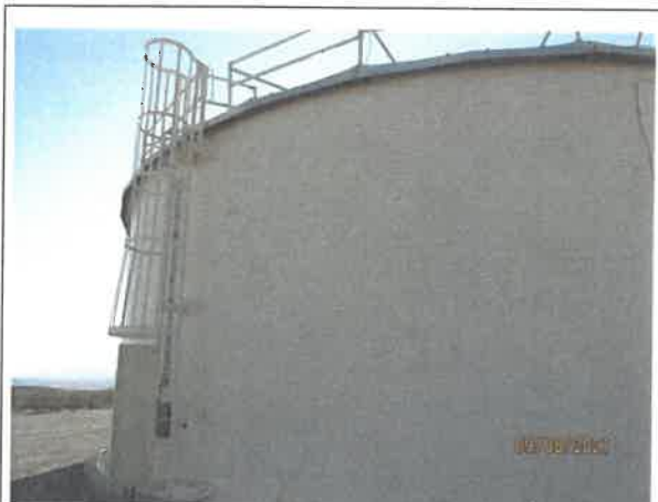
11 - Tank ladder with safety cage
