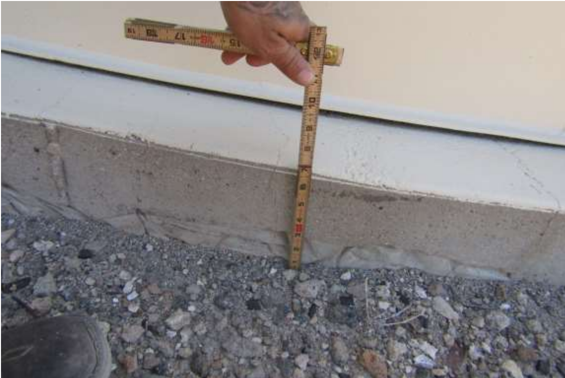
Photo shows the area around the tank foundation is properly graded and in compliance with AWWA D100-11; 12.7.1 Height aboveground.
