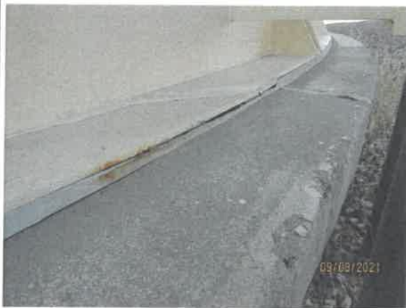
20 – Chime plate with minor corrosion and minor spalling for foundation
