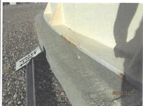
19 - Corrosion on chime plate
