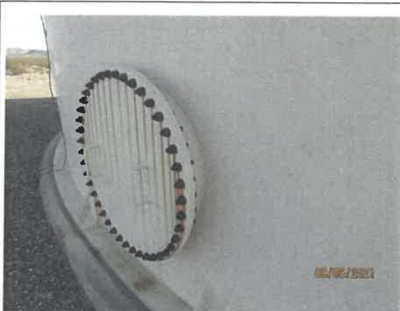
7 - Shell manhole with corrosion on bolts
