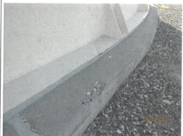
17 - Small spall on tank foundation
