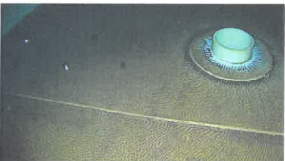
4:53 - Outlet pipe with sediment ring and dusting of sediment
