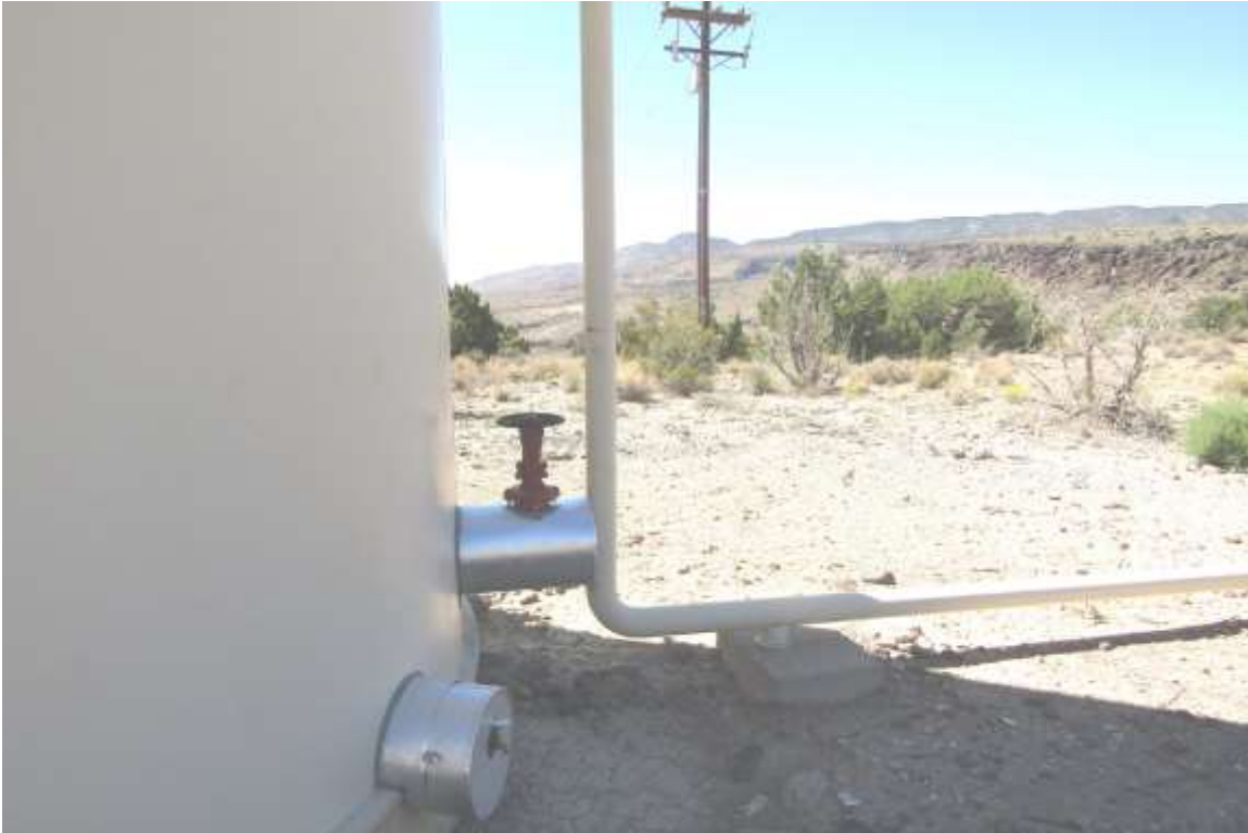
Photo shows the existing drain, which appears to be in good condition.
