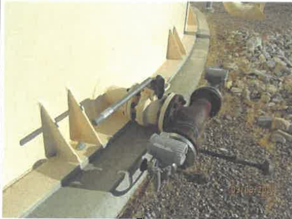
21 - Tank piping with sensors
