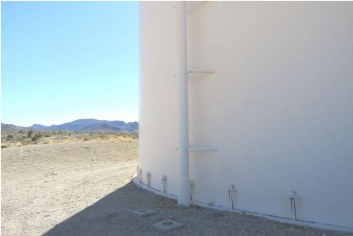
Photo shows the 12" overflow pipe system, which appears to be in good condition.
