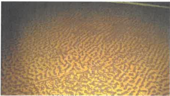
4:50 – Minor dusting of sediment on tank floor, coating is intact and free of corrosion
