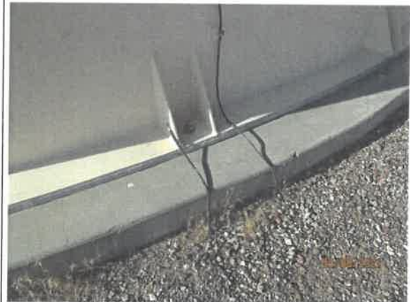
24 – Intact grounding wire
