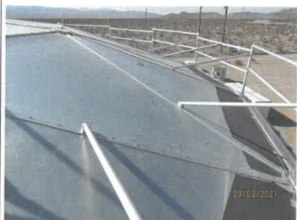
31 - Guardrails around 100% of roof
