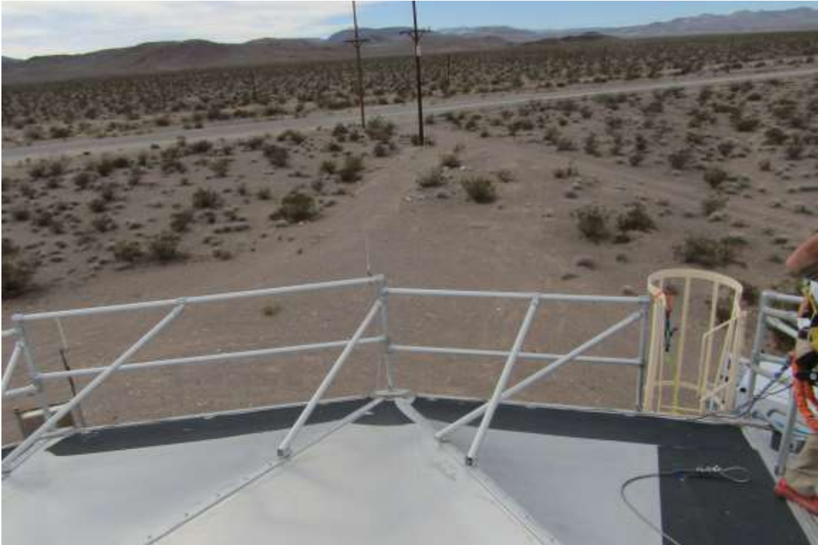
Photo shows the tank roof edge is equipped with a 38" high compliant handrail system for fall protection as required by OSHA 1910.28(b)(1) . The handrail system is equipped with an intermediate rail and toeboard.
