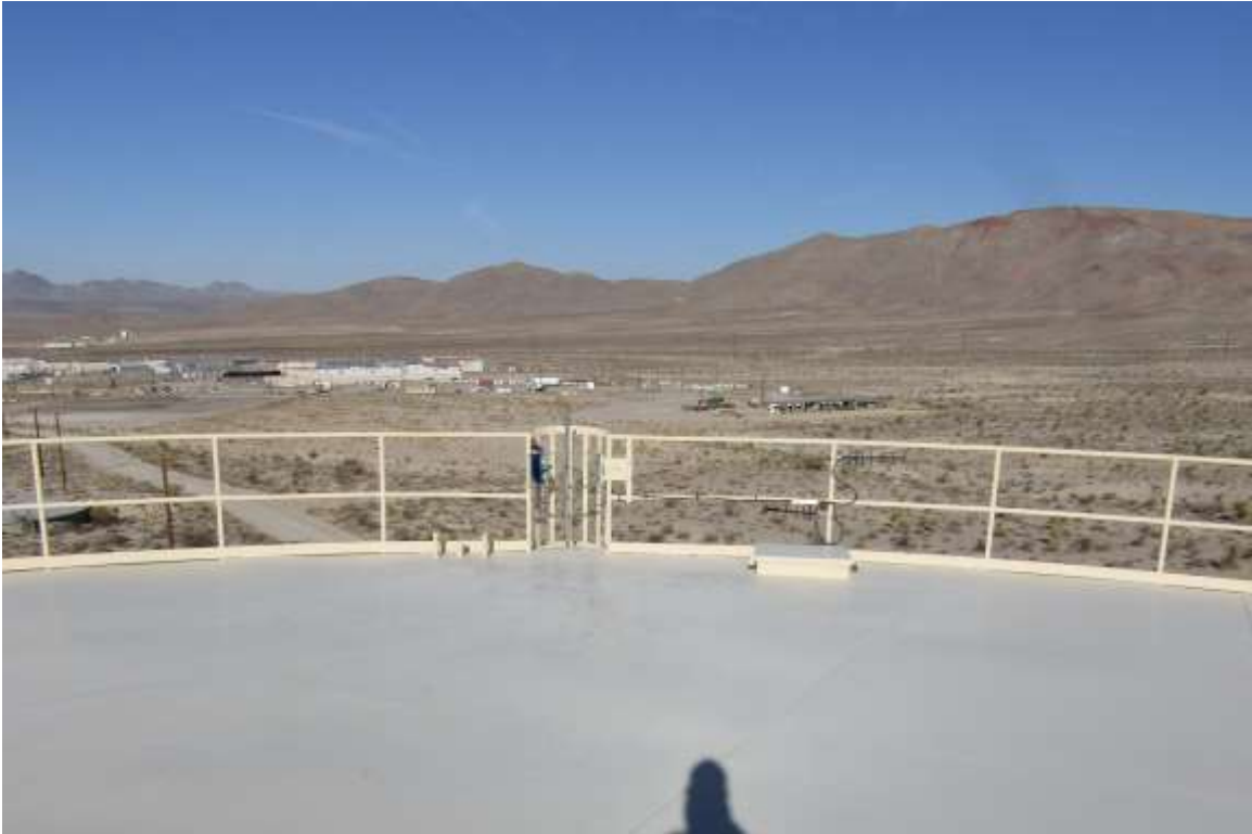
Photo shows the tank roof edge is equipped with a 42" high compliant handrail system for fall protection as required by OSHA 1910.28(b)(1) . The handrail system is equipped with an intermediate rail and toeboard.
