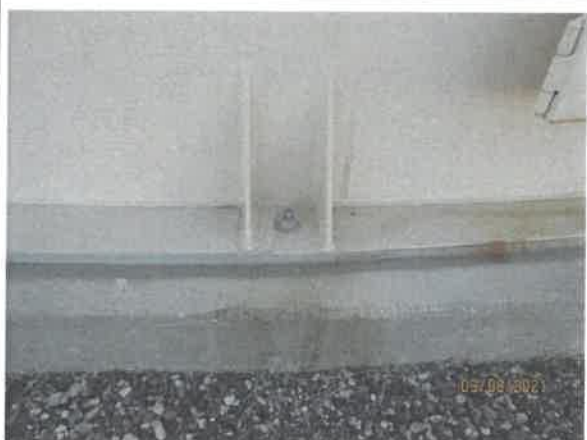
18 - Typical anchor bolt condition
