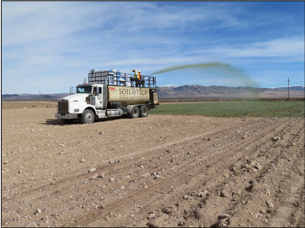
Figure 7-6. Applying Hydrostraw Guar Plus Formulation with a hydromulcher. (Photo taken February 13, 2024, by D.B. Hall)
