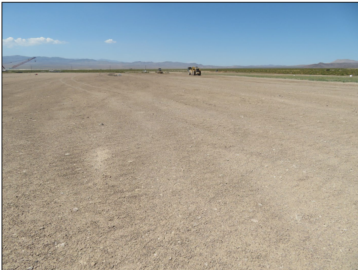
Figure 7-4. West Cover (CAU 111) under construction.
