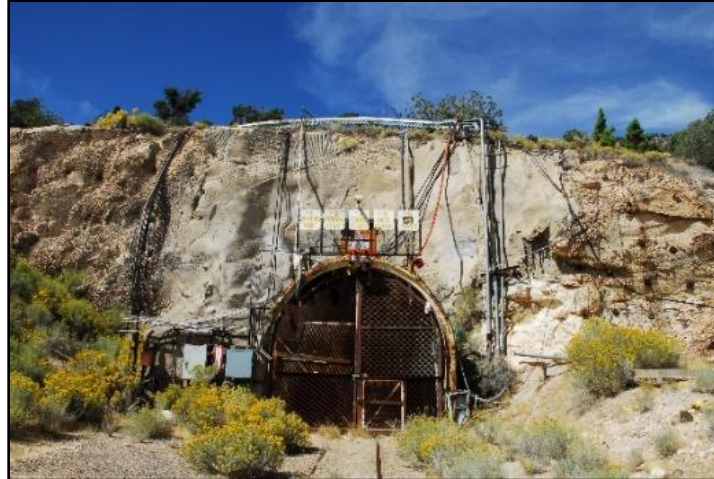
Figure F. 5 U12n Tunnel portal (DRI 2011).
