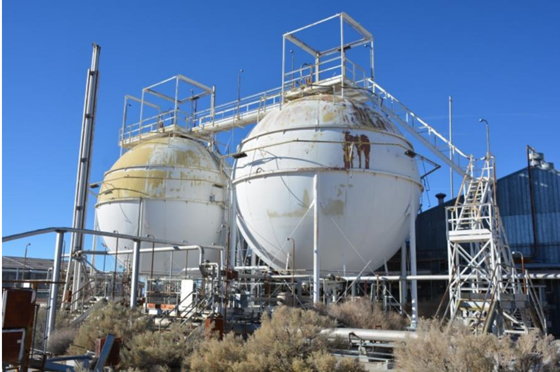
Figure B. 7 Test Cell C liquid hydrogen dewars at the NRDS (DRI 2019).
