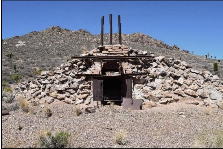
Figure B. 3 Mine Mountain stone-built lead and mercury retort (DRI 2018).
