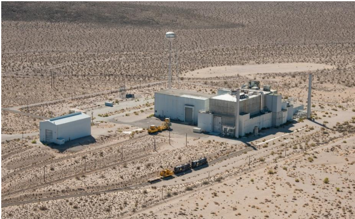
Figure B. 6 Overview of the Engine Maintenance and Disassembly facility at the NRDS (RSL 2013 D13_08081).
