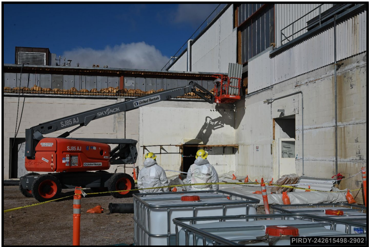
Workers removing galbestos paneling at EMAD Facility – February 2026
