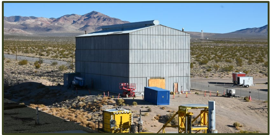
Above: A recent look at the trainshed at EMAD Facility.
