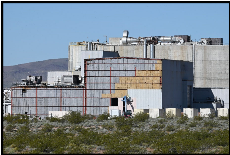
Below: Workers remove galbestos panels at EMAD Facility's Cold Bay – March 2026
