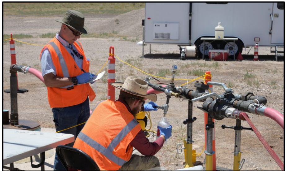
UGTA Team conducting pumping and sampling activities
