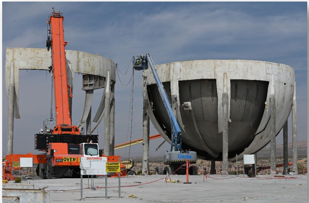
Hydrojet activities on the lower shells of Dewars 1 and 2 at TCC
