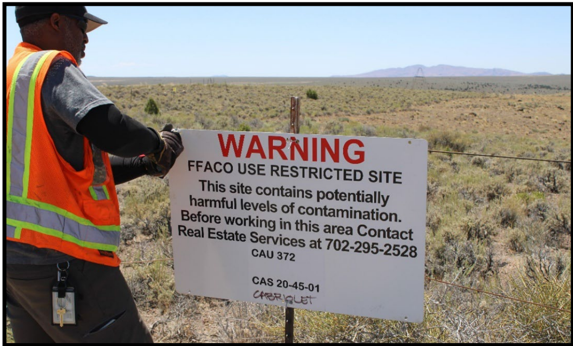
Photo above: EM Nevada Program contractor staff repair signs while performing post-closure inspections under the FFACO - July 2026
