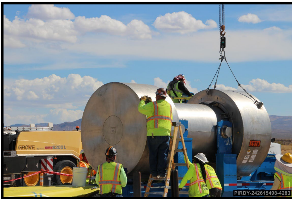
Photos at left and below: TVA baseplates unloaded and positioned for permanent disposal at the Area 5 RWMC - August 2026
