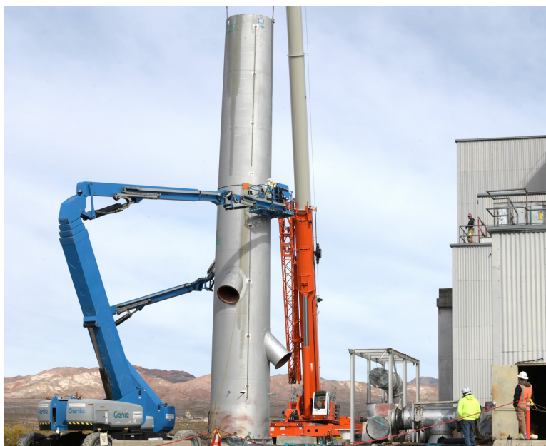
November 2024 demolition of an exhaust stack at the Engine Maintenance, Assembly, and Disassembly Facility
