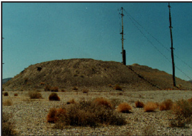
Gravel Gertie was instrumental in the design of the Pantex Plant in Texas and the Device Assembly Facility at the Nevada National Security Site.
